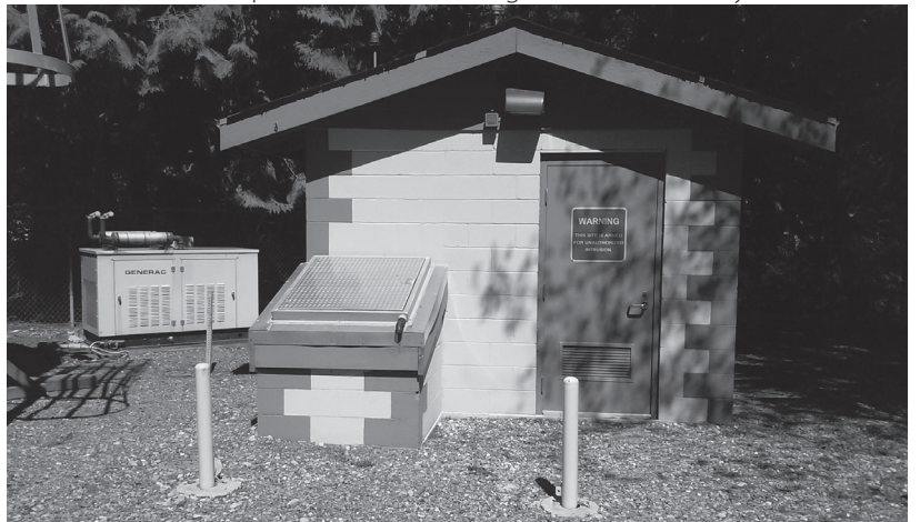
Braunwood Pump House
